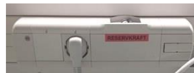
auxiliary electrical outlet on KB rail
