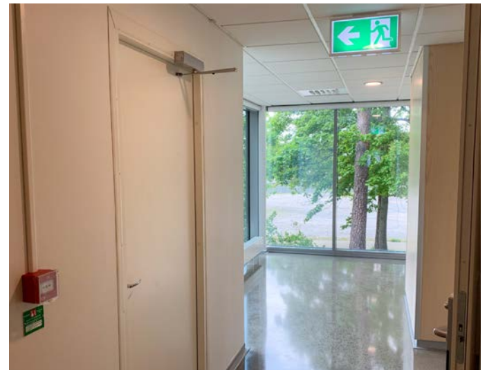
Picture of the door to the evacuation stairs
