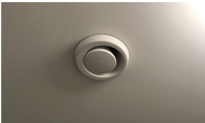
Ventilation in the bathroom
