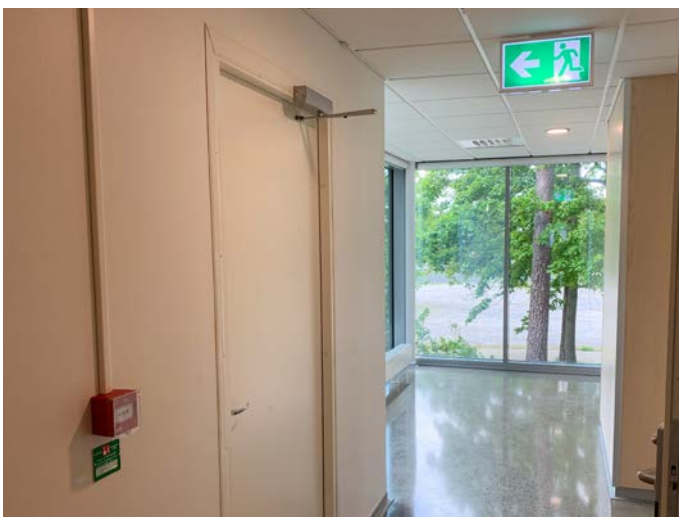
Picture of the door to the evacuation stairs and the emergency exit.
